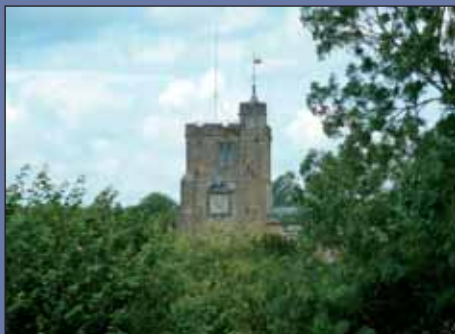
Cranbrook's St Dunstan's Church Tower
